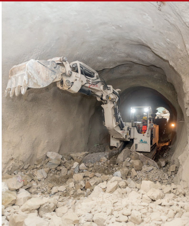
Tunnel loading machines
